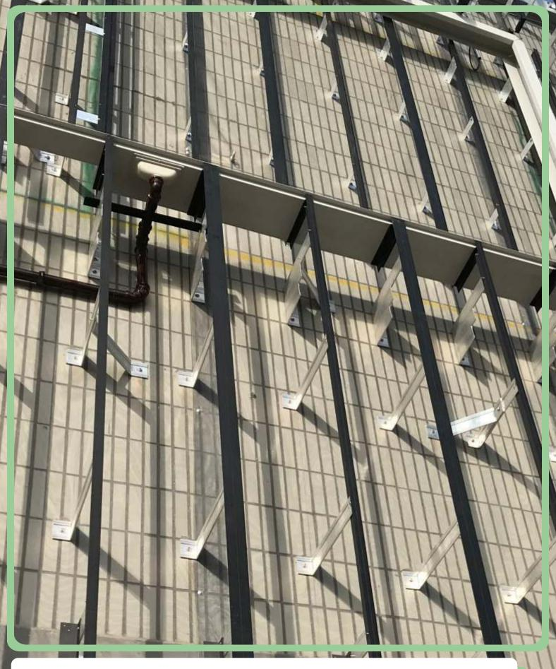
This illustrates the technical solution adopted for irregular spacing, using custom elements and brackets dimensioned according to their function. All include slotted holes; support brackets are combined in threes to form a diagonal brace, and bracing bars ensure structural stability. This demonstrates a high-performance technical solution, reflecting solid engineering, sound judgment, and a commitment to the quality and safety of ventilated façades.
