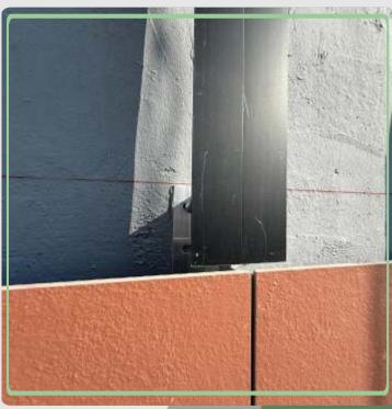
This shows cladding installation perfectly aligned with the profile face, while properly respecting expansion joints. This step is fundamental to absorbing thermal movement and ensuring system durability. Ventilated façade execution demands refined technique, strict dimensional control, and full compliance with construction standards. It is a system that does not allow improvisation and requires precision in every detail to ensure performance and stability.
