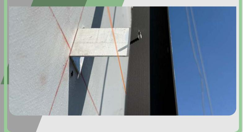
In this case, the alignment string was properly placed at the rear of the profile, where the support point is minimal just 2.5 mm and free from interference caused by possible flange inclinations. Once the cladding is applied, flatness will be naturally preserved, since alignment was based on the spine of the profile. This mounting technique exemplifies good construction practices and reflects a technical rigor that directly supports system performance and durability.
