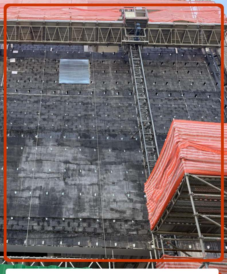
A lack of standardization is observed in the installation of brackets, with a reduced height of 10 cm and fixation by a single anchoring point, limiting their structural capacity. Additionally, extensions are used to compensate for spacing, reusing the same vertical profile screwed onto the base bracket. This configuration goes against good design practices and may compromise the stability of the system, increasing the risk of structural failure.
