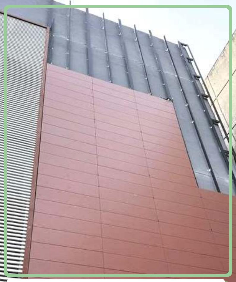
In this case, a 300×1200×10 mm cladding panel was installed. Despite its high flexural strength, its smaller size prevents it from being affected by system-induced tensions. We also use 1000×3000×3 mm panels in our portfolio, which due to their low flexural stiffness can absorb deformations and accommodate movements. Each format behaves differently and must be evaluated according to the project demands and façade dynamics.
