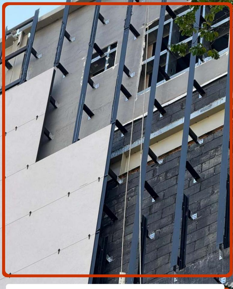
A combination of solutions contrary to established technical principles is seen. Significant bracket extensions with T-profiles are present, apparently without structural calculation support. Furthermore, the lack of bracing and the presence of fixations acting as rigid joints generate unwanted tensions. These conditions reveal critical weaknesses and, in our view, may represent risks to the stability of the façade and the safety of the building.
