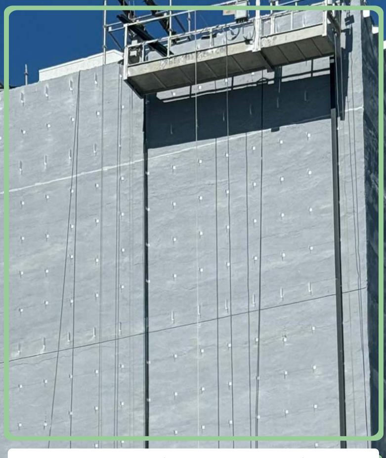
Brackets measuring 18 cm with two anchors for support and 6 cm with a single anchor for retention are used. These are single pieces, precisely positioned to match the spacing of the layout and the correct heights for fixing the vertical profiles. The execution demonstrates a defined technical design, with pre-specified anchoring points and strict dimensional control a critical condition for the system's performance and stability.
