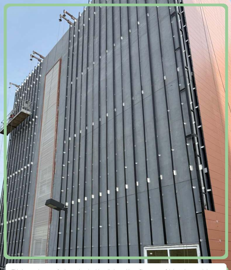
This image shows perfectly synchronized installation, with profiles custom-fabricated to match beams and align with cladding joints. Each profile starts and ends exactly at the bracket, following parameters defined in the design. This fully controlled execution demonstrates technical planning, dimensional precision, and attention to detail. Such control is essential to ensure system stability, material durability, and the final quality of the ventilated façade.
