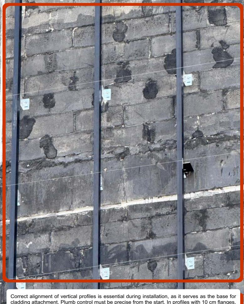
Correct alignment of vertical profiles is essential during installation, as it serves as the base for cladding attachment. Plumb control must be precise from the start. In profiles with 10 cm flanges, using the front face as a guide may cause millimetric deviations which, when accumulated, compromise the geometry, flatness, and finish of the façade.
