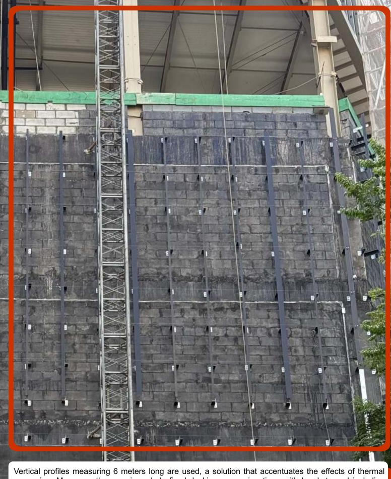
Vertical profiles measuring 6 meters long are used, a solution that accentuates the effects of thermal expansion. Moreover, they are irregularly fixed, lacking proper junctions with brackets and including cantilevered segments. Many remain attached with screws into profile T extensions, acting as rigid links. This configuration restricts the natural movement of components, favoring internal stresses that may cause deformation, detachment, or failure of the cladding.
