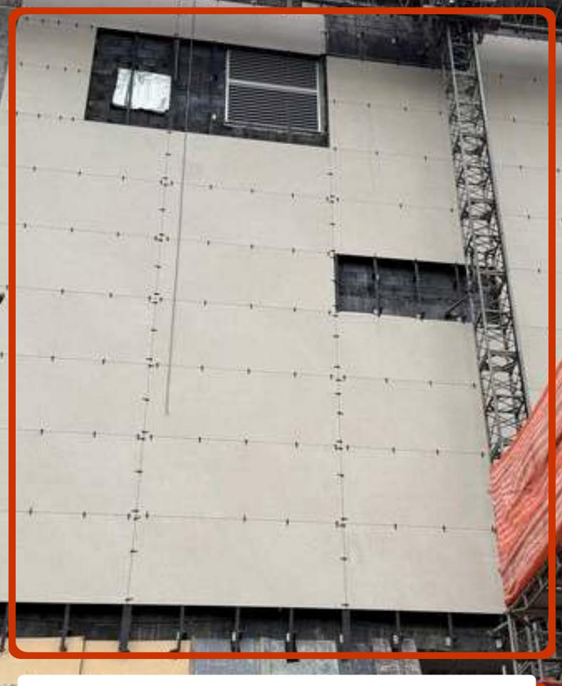
Applying a 1200×2800×6 mm cladding panel highly rigid and resistant to flexing directly onto profiles is technically critical. Being a large-format piece with low deformation tolerance, its installation requires continuous support and tension relief mechanisms. Failing to meet these criteria can undermine performance and significantly increase the risk of failure by breakage or detachment over time.
