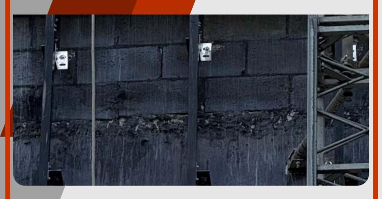
The situation observed raises serious technical concerns. Six-meter vertical profiles already a sensitive solution were joined using angle brackets to form 12-meter linear elements, with no apparent provision for thermal expansion. This practice ignores fundamental principles of thermal control and structural stability, potentially compromising system performance. The lack of proper joints can lead to irreversible deformations and risk the integrity of the façade.
