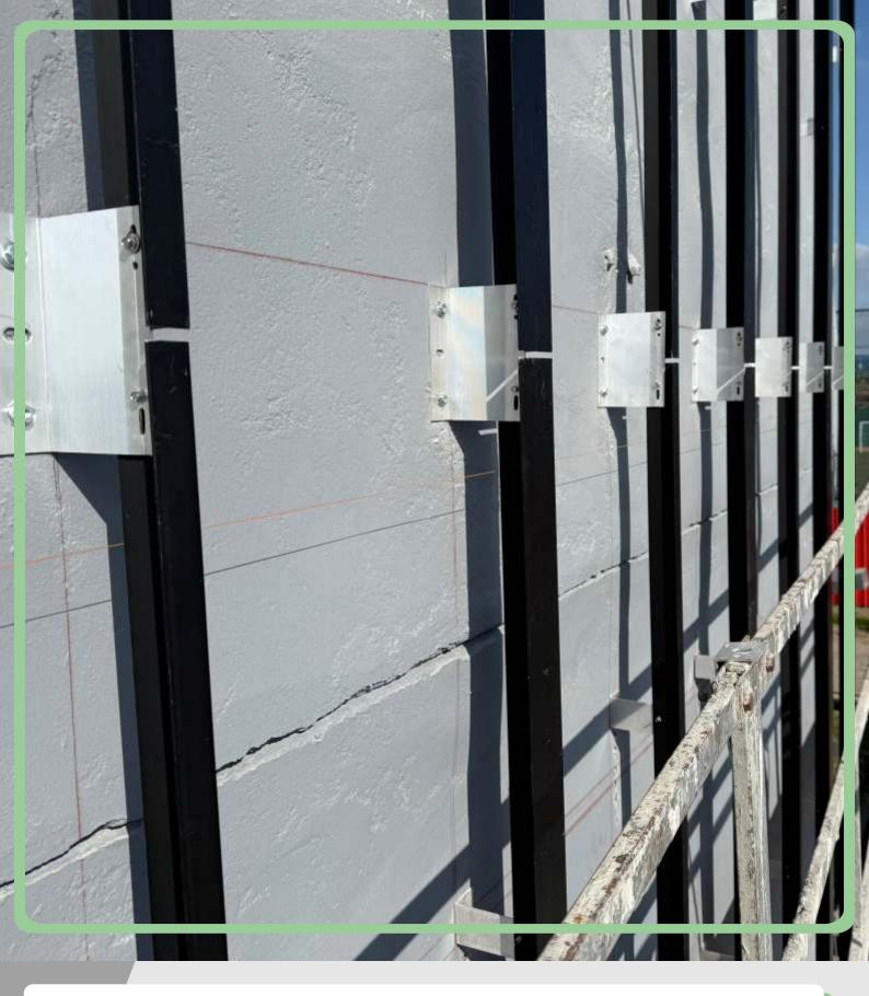
The 10 mm joint was correctly applied, in compliance with technical expansion standards. The vertical profile was fixed as a rigid point at the top and as a sliding point at the bottom, allowing the system to properly respond to thermal and structural movement. This is a clear example of well-planned technical execution, aligned with engineering best practices and optimization of anchoring and fixing elements, ensuring safety and durability.
