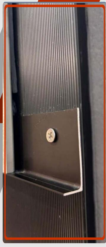
Grooves were designed to increase the contact surface between the MS polymer and the substrate. However, technical studies and field observations show this method may complicate application. The adhesive often fails to fill the grooves uniformly, promoting voids and air bubbles. This compromises the regularity of the adhesive bead and makes cleaning more difficult. As a result, this practice is gradually being phased out in technically demanding applications.
