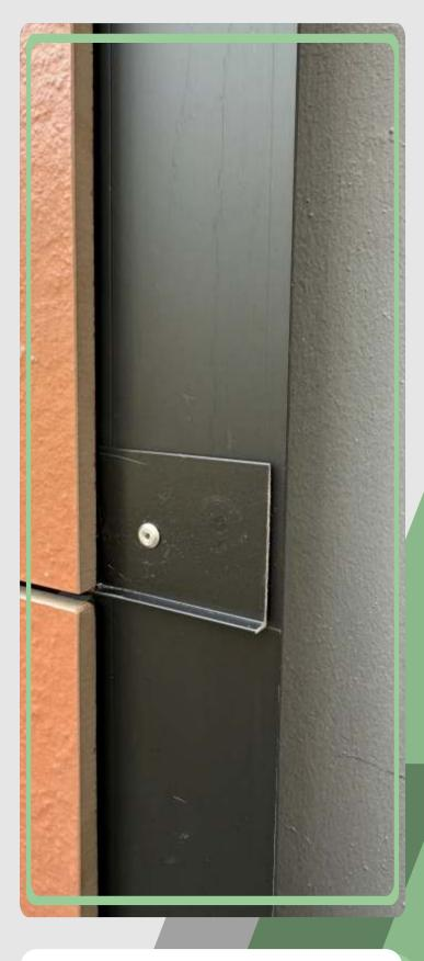
A smooth surface offers ideal conditions for MS polymer application. Being regular and continuous, it allows the adhesive to spread uniformly, forming a cohesive layer without internal defects. This ensures a consistent bead thickness, essential for proper curing and structural performance. It also improves cleaning by eliminating dust and debris, and enhances the micro-suction effect, contributing to better adhesion.
